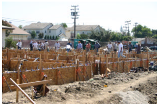
Construction begins on the FCSN "Dream Center"
